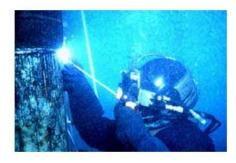
In wet welding MMA (manual metal arc welding) is used.
